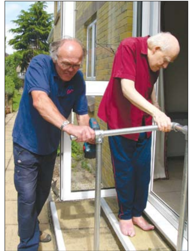
Handrails can help prevent falls
